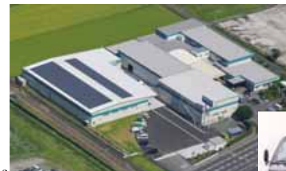
Install solar panels
